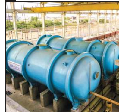
Sand Filter Tanks for Bandar Abbas Desalination Project
