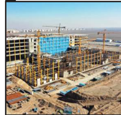
Steel framework of Block C of Khatam Qom Hospital
