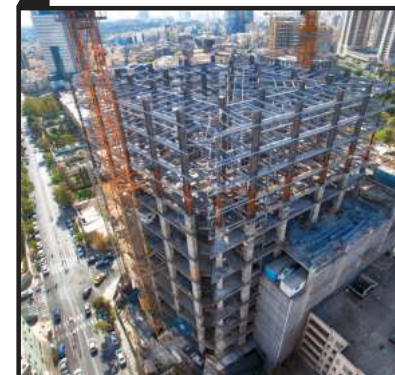
Steel framework for the Metal Hotel project
